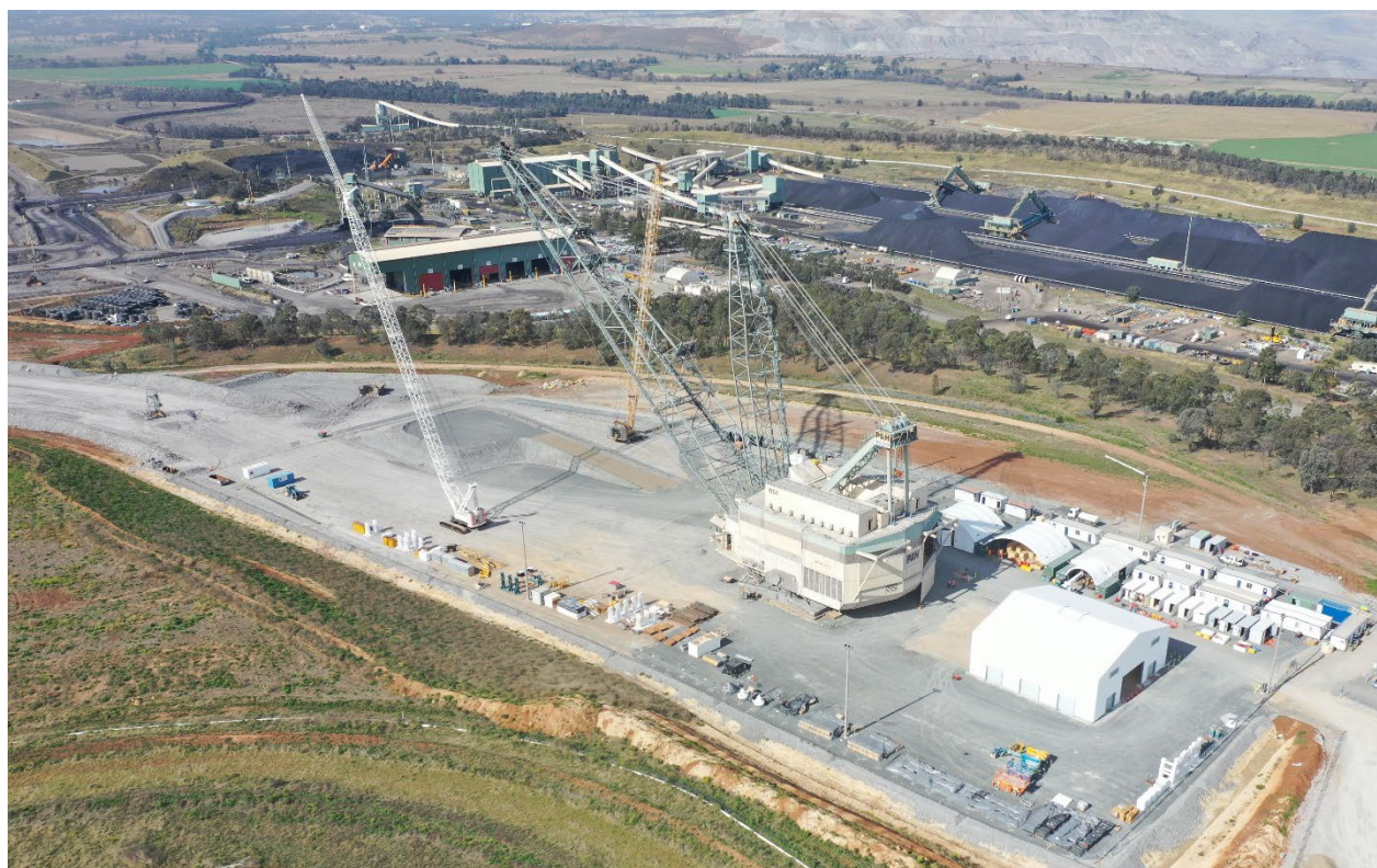
Aerial view of the Bengalla dragline under maintenance.
